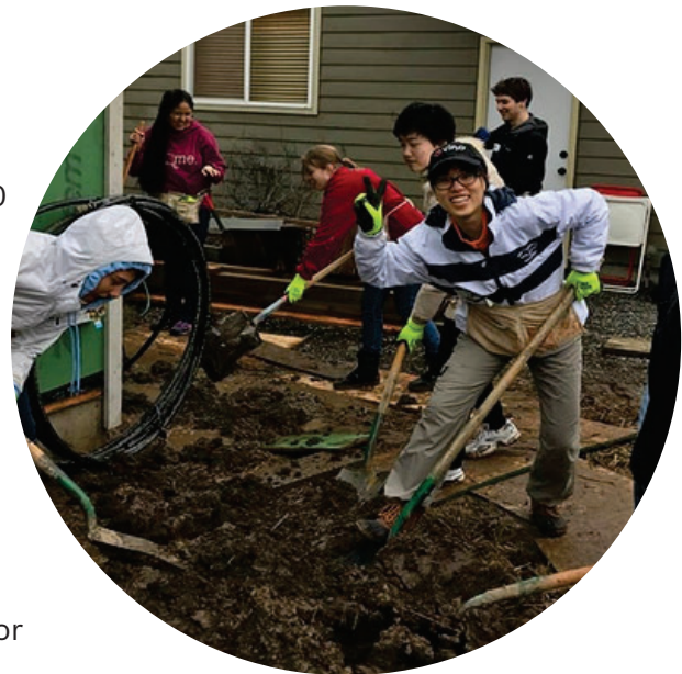
Students building and digging in front of Habitat for Humanity project
